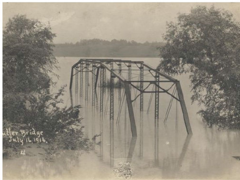
Butler Bridge in Asheville was covered by the flooding of the French Broad River in July 1916. (Photo: Citizen-Times photo)
